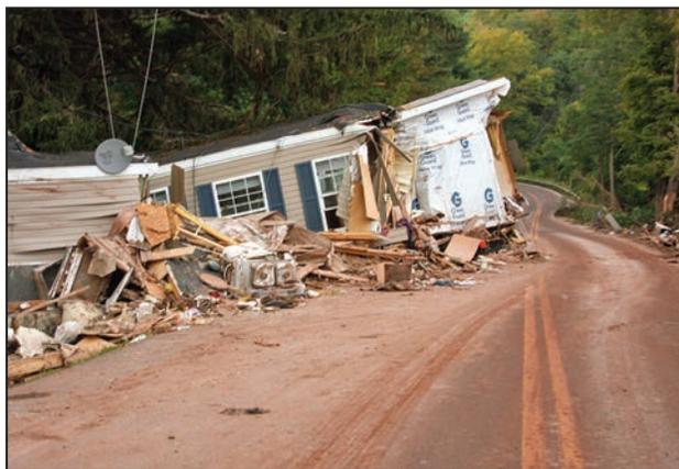
**A flooded manufactured home can float off its foundation and cause additional damage nearby.**
